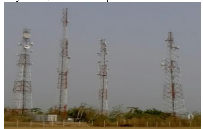
Figure 3. Base Transceiver Station (BTS) of the Service Providers
