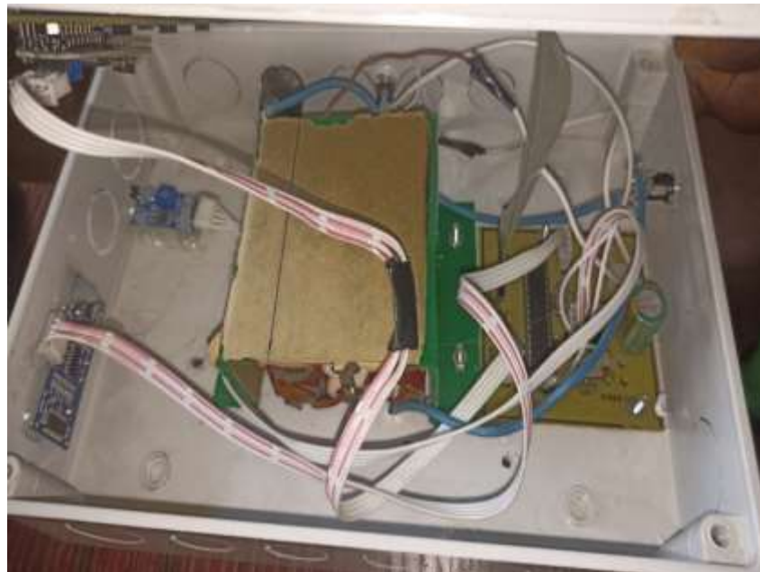
Figure 4: Fabricated illustrations of the speed detection and measurement system.
